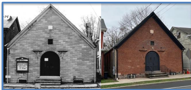
Historic Structures Survey left; author's March 2024 photo right shows the stone face "improvement" removed and provides a semblance of its original appearance.
